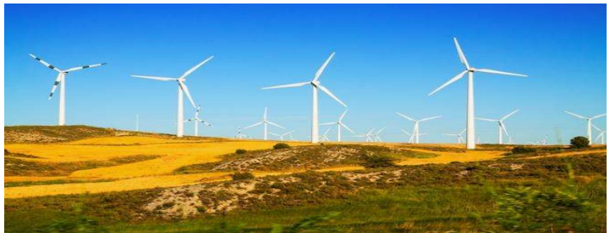
Figure 12. Onshore wind farms.
